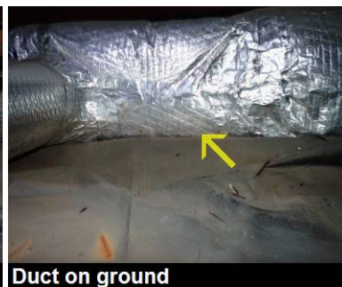
Duct on ground
