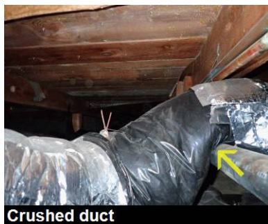
Crushed duct
