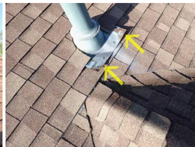
Flashing lifting
