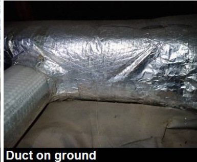
Duct on ground
