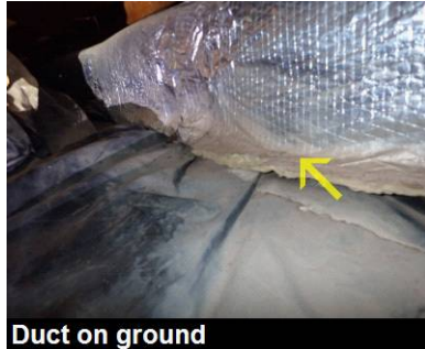
Duct on ground
