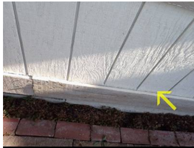
Flashing missing
