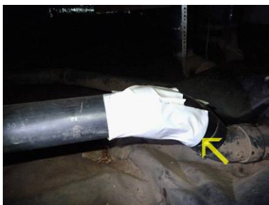
Substandard repair
